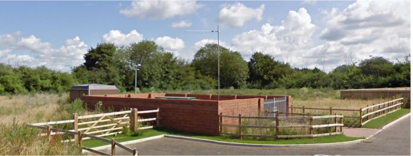
figure 6: Existing pumping station and enclosure surrounded by application site
