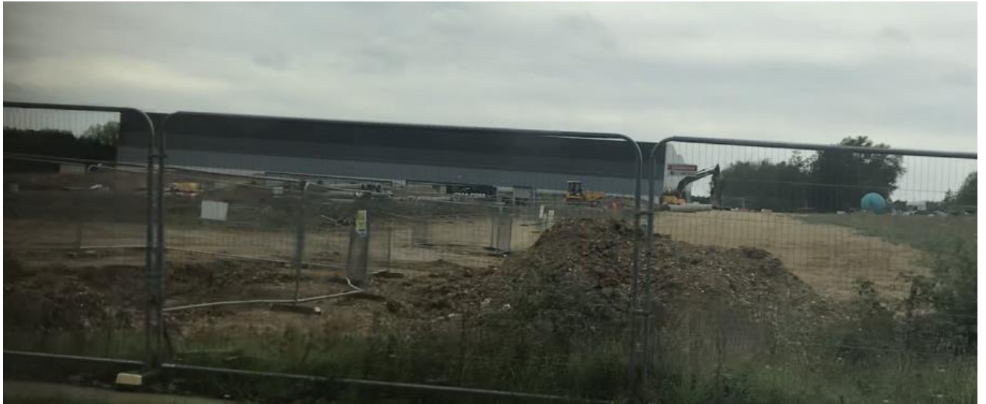
Figure 2. Approved Scheme Currently Under Construction
